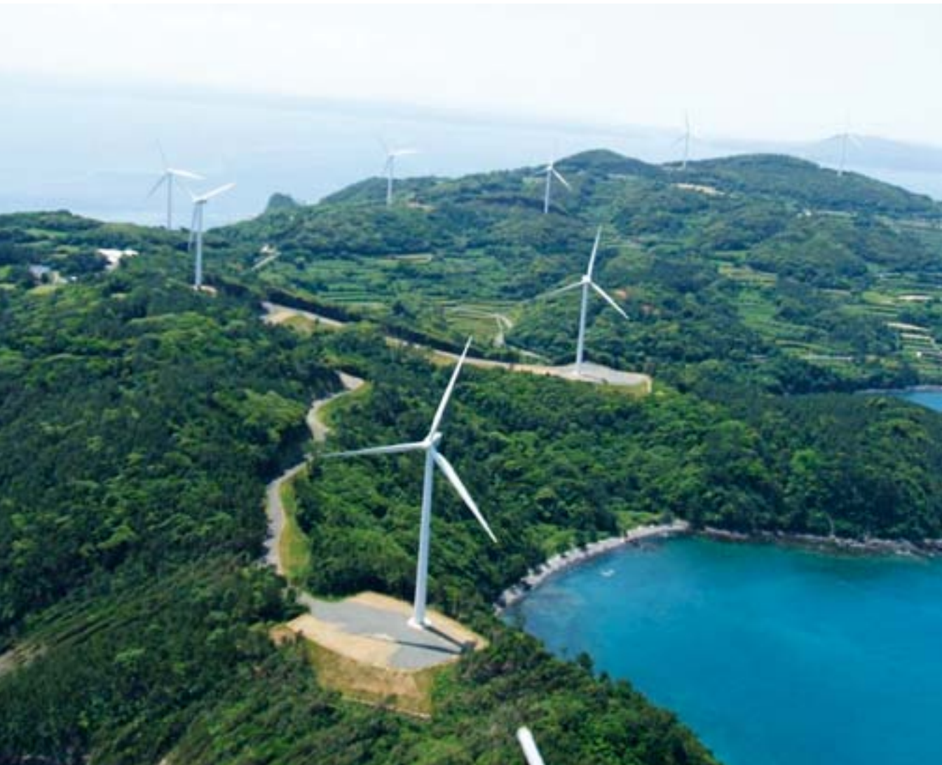
Azuchi Oshima wind farm, Nagasaki, Japan © M&D Greenenergy Co. Ltd
