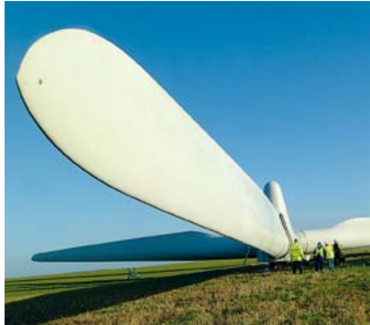
Blades ready for lifting', Out Newton, UK © EON
