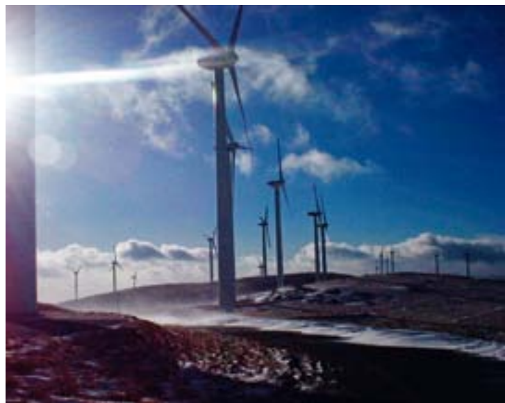
Kamaishi Wind farm, Japan © M&D Green Energy Co. Ltd.
